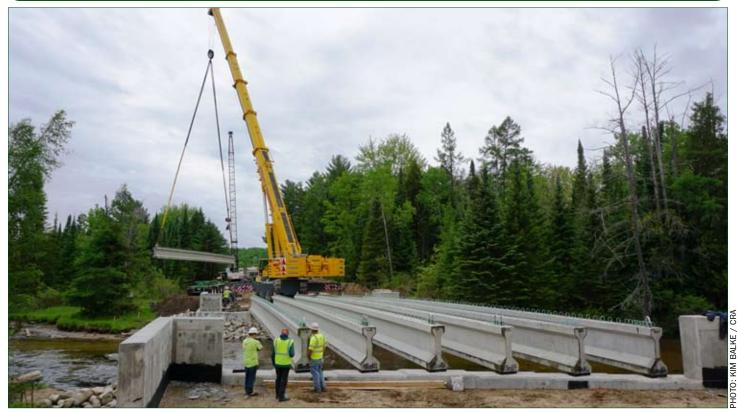
NEARING COMPLETION. Work continues on the new Chestonia Bridge over the Jordan River at Old State Rd. with the laying of seven reinforced concrete beams the end of May. The \$1.27 million dollar project, begun the end of February, replaces two aging, undersized culverts with a clear span concrete bridge, marking a milestone in restoring the Jordan to a free flowing river. Construction is being handled through the Antrim County Road Commission, following a
